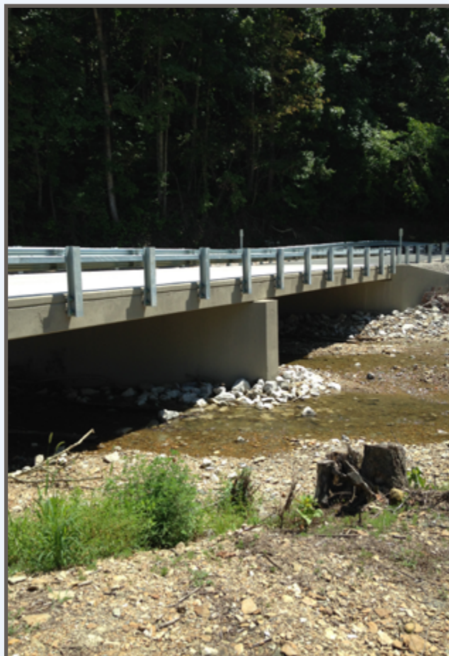
Bridge over Brush Creek in Casey County
